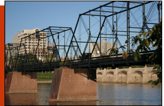
Walnut Street Bridge
