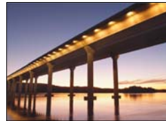
Multi-Span Category I-76, Susquehanna River Bridge – Submitted by FIGG
